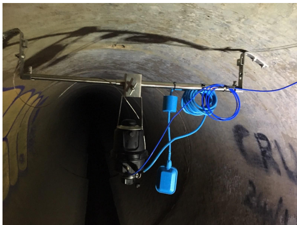
Pollution monitoring equipment installed in stormwater drains
